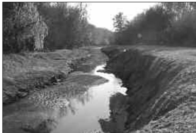
The upper reach of Tumblin Creek is restricted within a narrow channel and spoil pile berm that isolates the floodplain to the west (right) of the berm from more frequent flooding.
