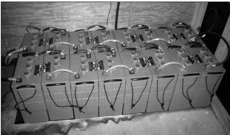
Sixteen deep-cycle batteries for storage of energy generated by solar panels.
