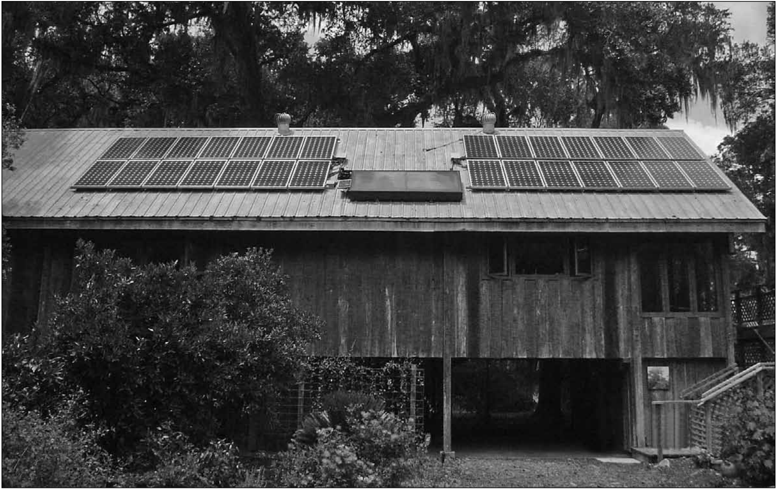
New solar panels on the home of Josh and Sally Dickinson.
